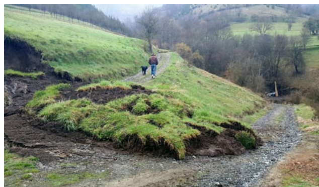
Picture 2: Municipal macadam and dirt roads in Kraljevo Municipality damaged by landslides (source: www.kraljevo.biz )
