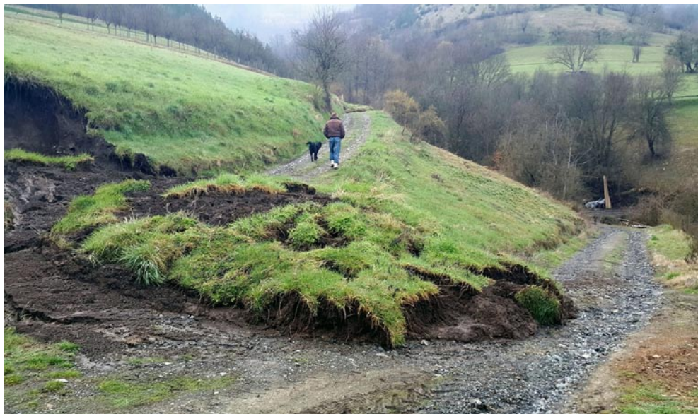
Picture 2: Municipal macadam and dirt roads in Kraljevo Municipality damaged by landslides (source: www.kraljevo.biz )
